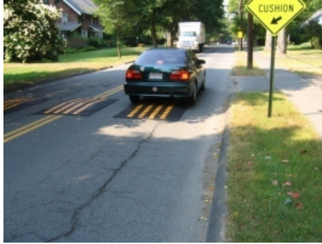
Figure 50 Vehicle straddling the smaller speed cushions
