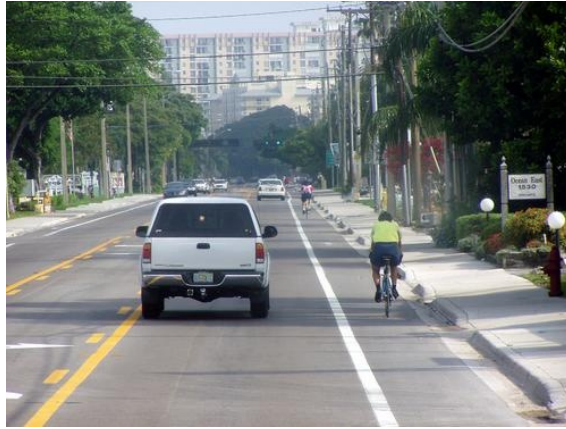
Figure 33 A converted four-lane roadway to three-lane roadway (44)
