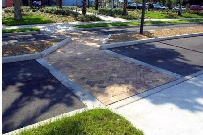
Figure 39 Pedestrian crossing island with angled crosswalk (44)
