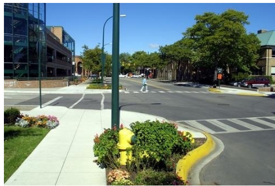
Figure 36 Curb extensions at an intersection (44)
