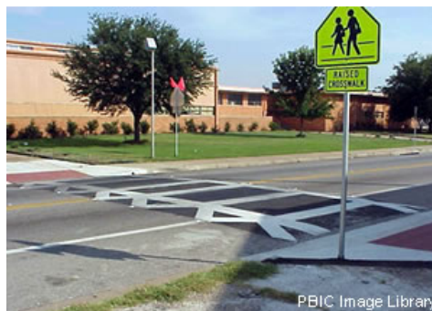
Figure 26 Permanent speed table/raised crosswalk (38)
