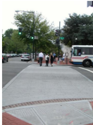
Figure 35 Stamped concrete pedestrian crossing (44)
