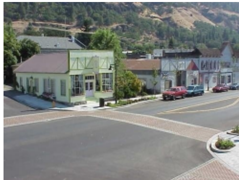
Figure 37 Intersection bulbouts at an intersection (44)
