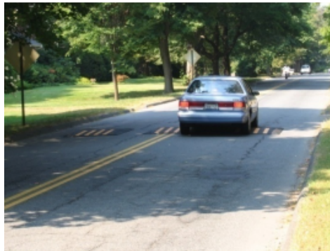
Figure 51 Vehicle forced to decrease speed due to speed cushions
