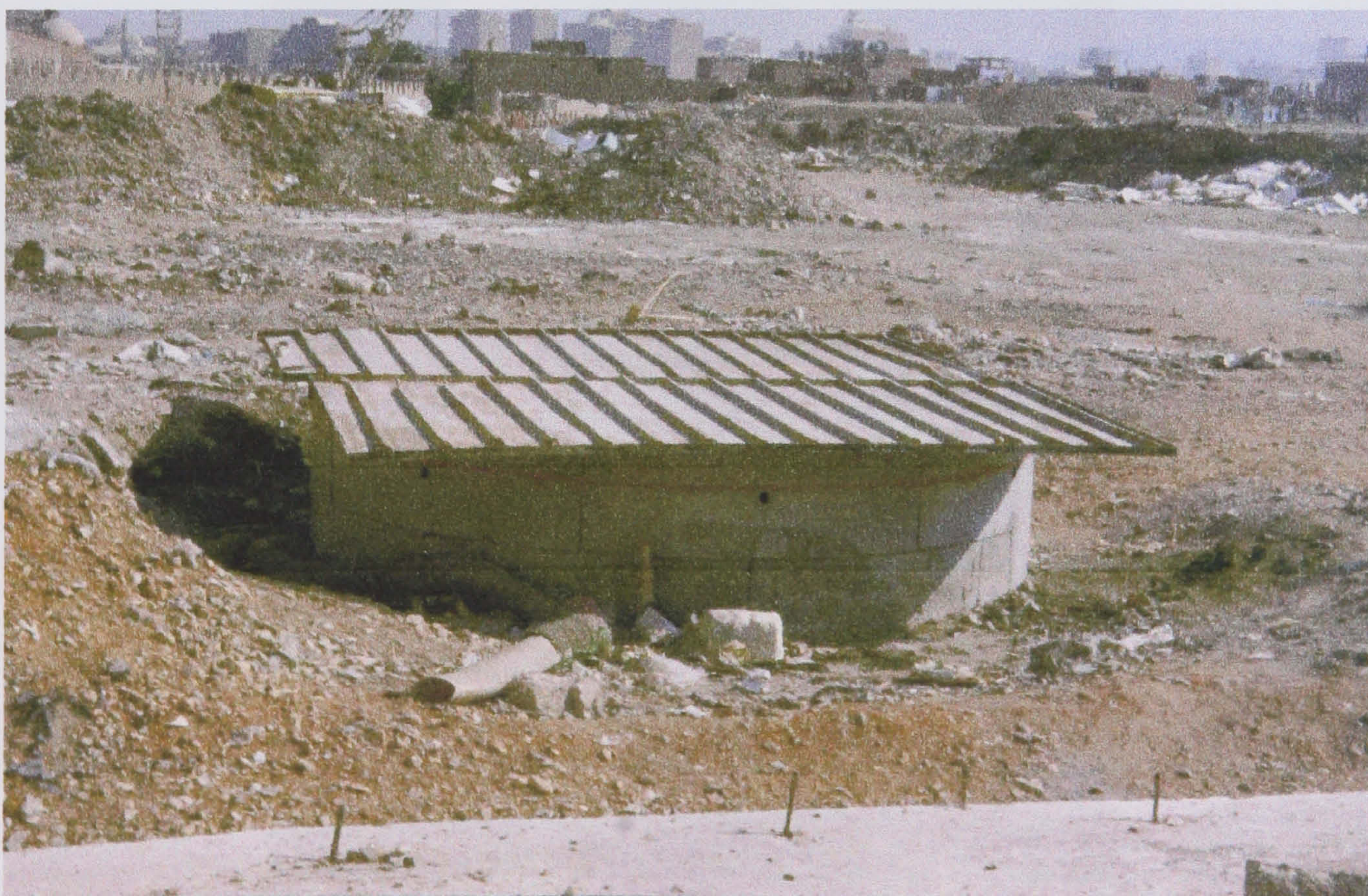
B: View of shaft 6 with the wall of the Mosque of 'Amr in the top left corner.
