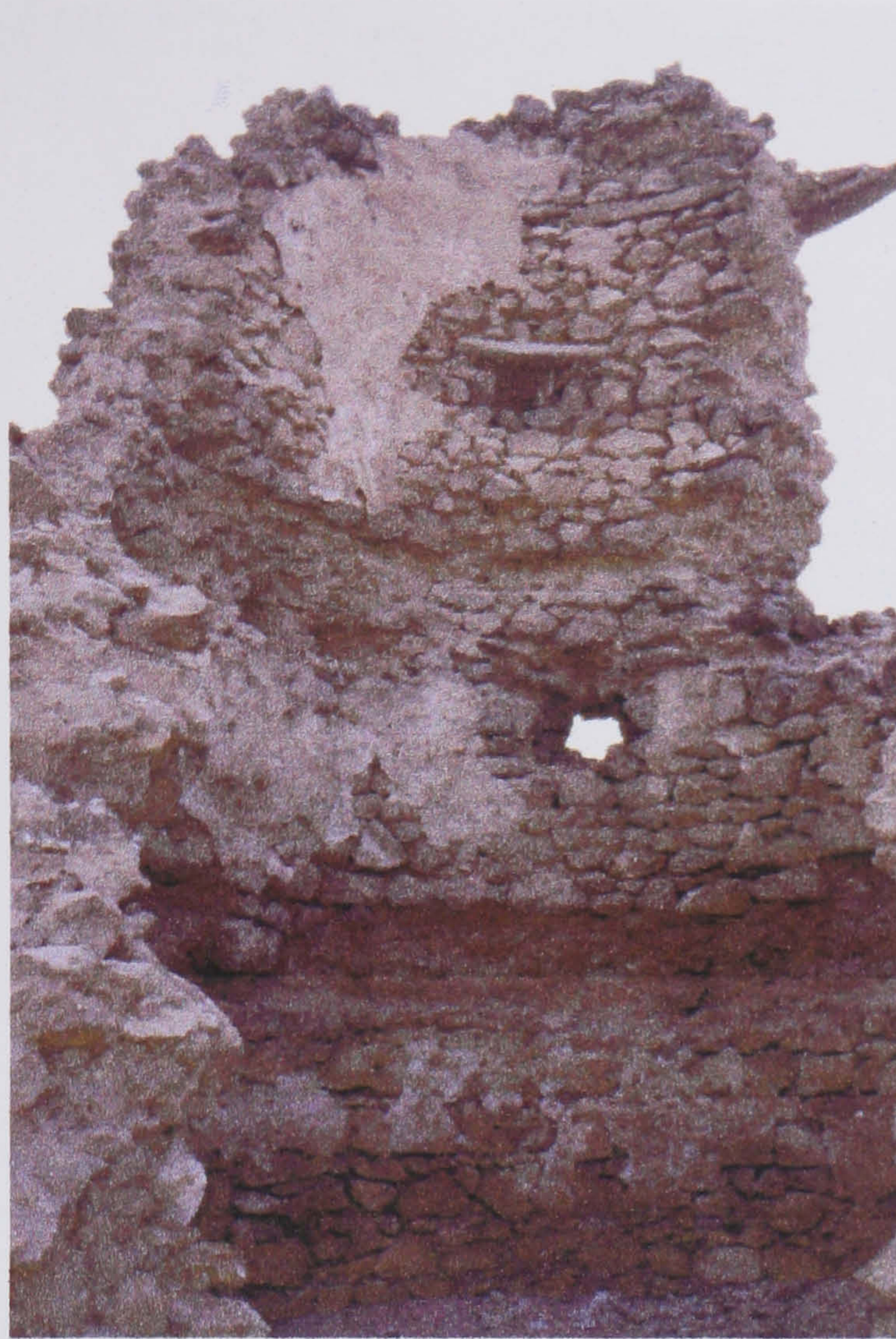
A: Interior of watchtower.
