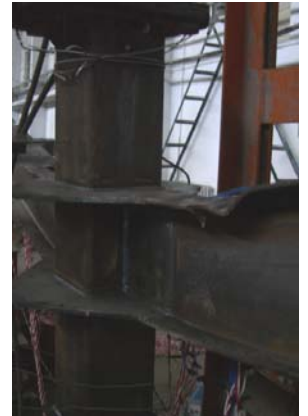
(e) Buckling of beam in joint C
