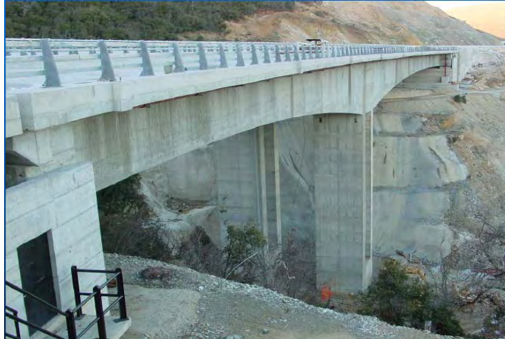
Figure 2.1: View of Polymylos bridge
