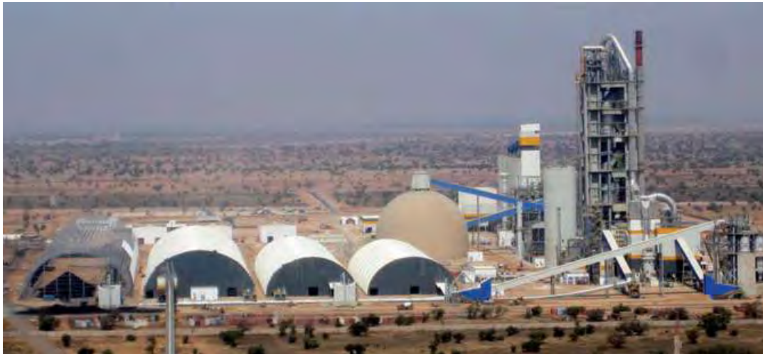
Figure 1.3: Italcementi's Ait Baha plant in Morocco
