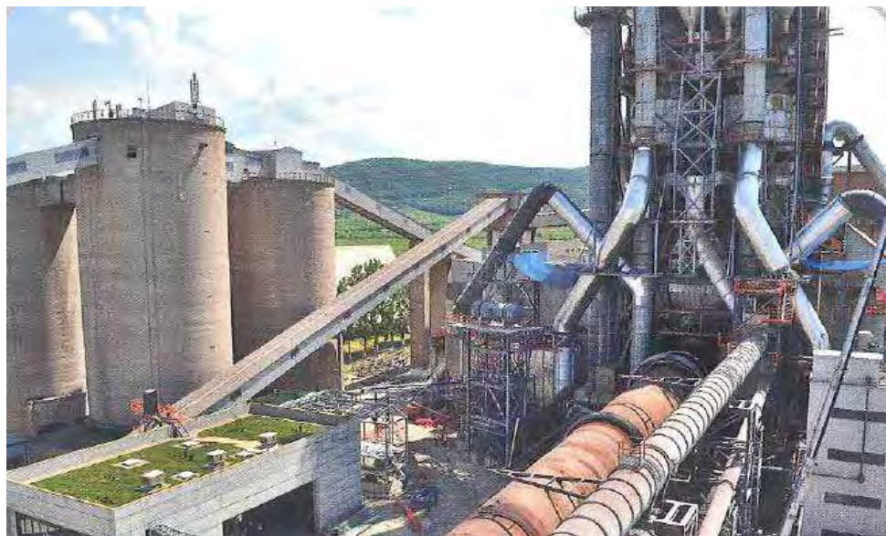
Figure 1.5: Holcim Alesd cement plant – Romania
