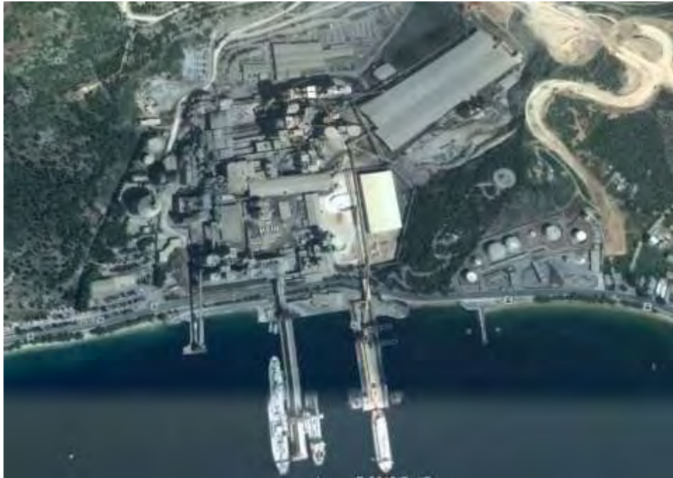
Figure 2.2: Volos cement plant
