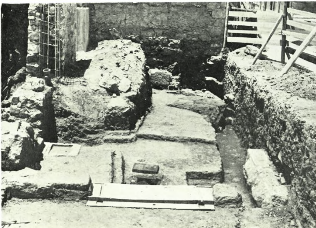
Athens, Artemis Aristoboule: a. General View of Temple from Southwest, b. General View of Excavation from East
