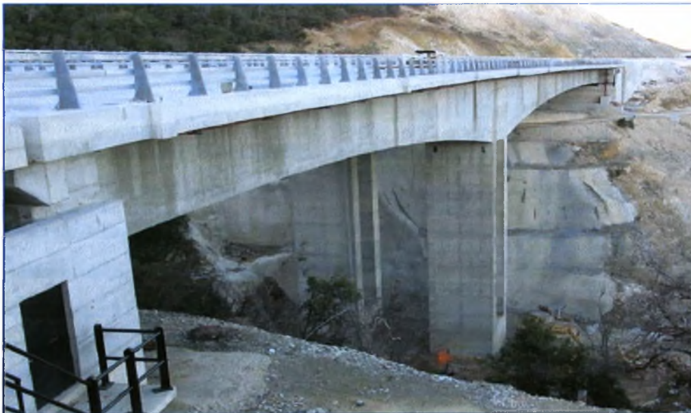
Figure 5.24: View of 9 th Polymylos bridge
