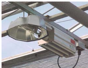
Figure 7.5 Selected lamp with attached ballast for HPC prototype.
