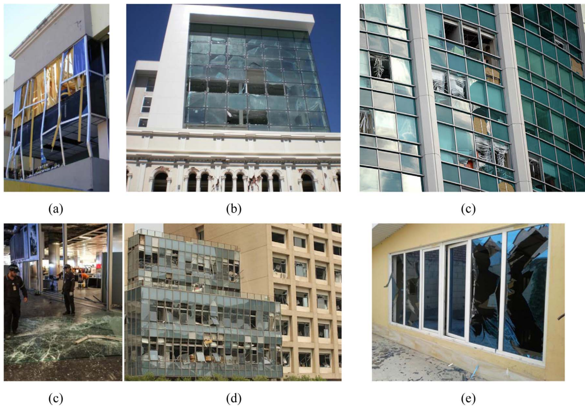
Fig. 2. Examples of glass systems under hazards: (a)–(b) seismic events, (c) hurricanes and (d)–(e) explosions.
