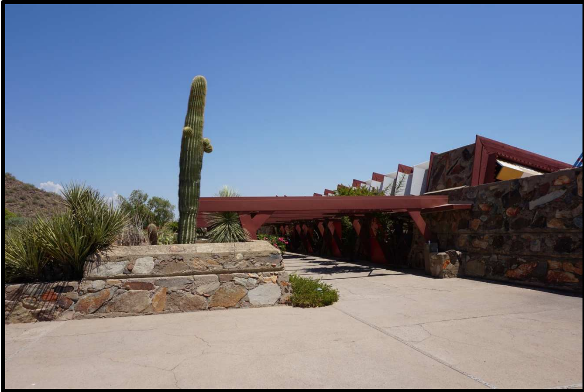
Figure 4.8. Repeating crossbeams above the main axis create clear, discernable, and accentuated transitional space , and provide a connection and coherence as referred in organized complexity ‘attribution’ of biophilic space and place experience .
