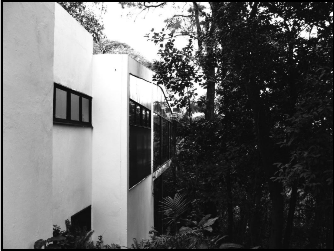
Figure 4.30. Glass House reflects a synthesis of modern and vernacular from the different stylized front and back façades.
