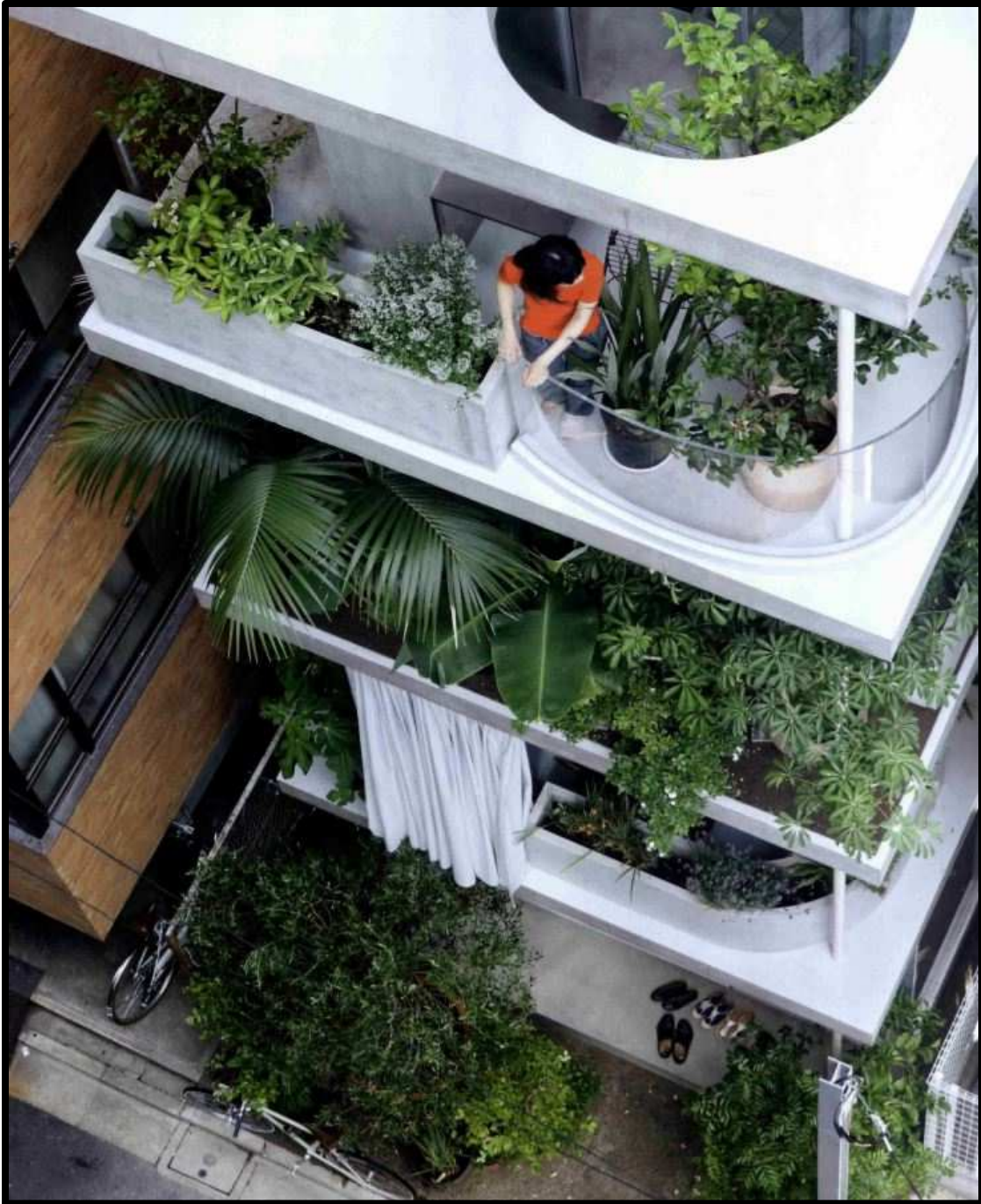
Figure 4.40. The green façade of Garden & House proposes an open life style. Reprinted from “Jardin y casa = Garden & House, 2006-2011, (Japan/Japan): [Office of Ryue Nishizawa],” 2015-01-01, AV Monografias, AV Monographs , 171-172, p. 175. Copyrights 2011 by Iwan Baan, and 2015 by AV Monografias, AV Monographs.
