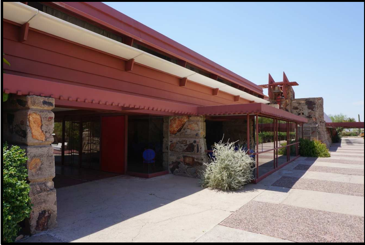
Figure 4.19. The Dining Room and breezeway adjacent to the Drafting studio.
