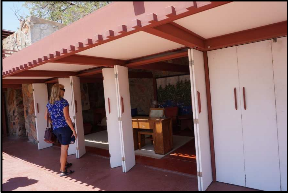
Figure 4.16.a. Wright's Living Quarter's operable doors apply the biophilic experience of space and place by the direct experience of nature on the site.
