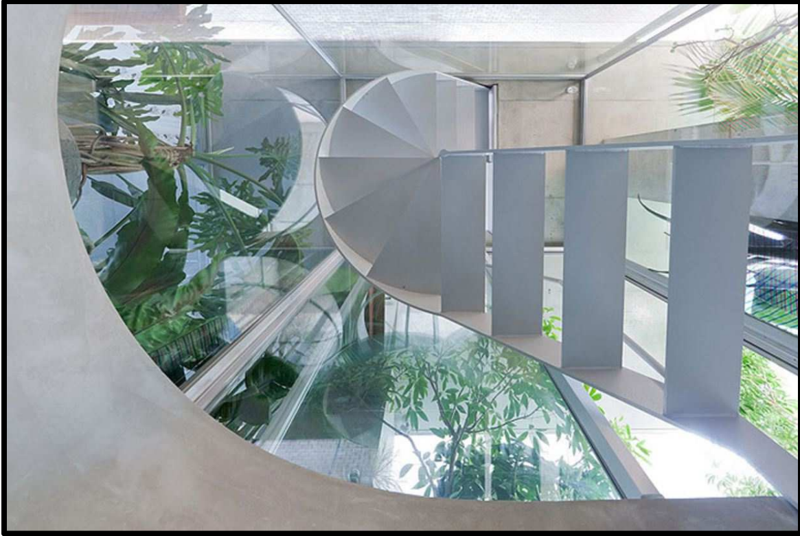
Figure 4.43. The unique architectural promenade of the house is set by a steel custom made white painted spiral staircase.
