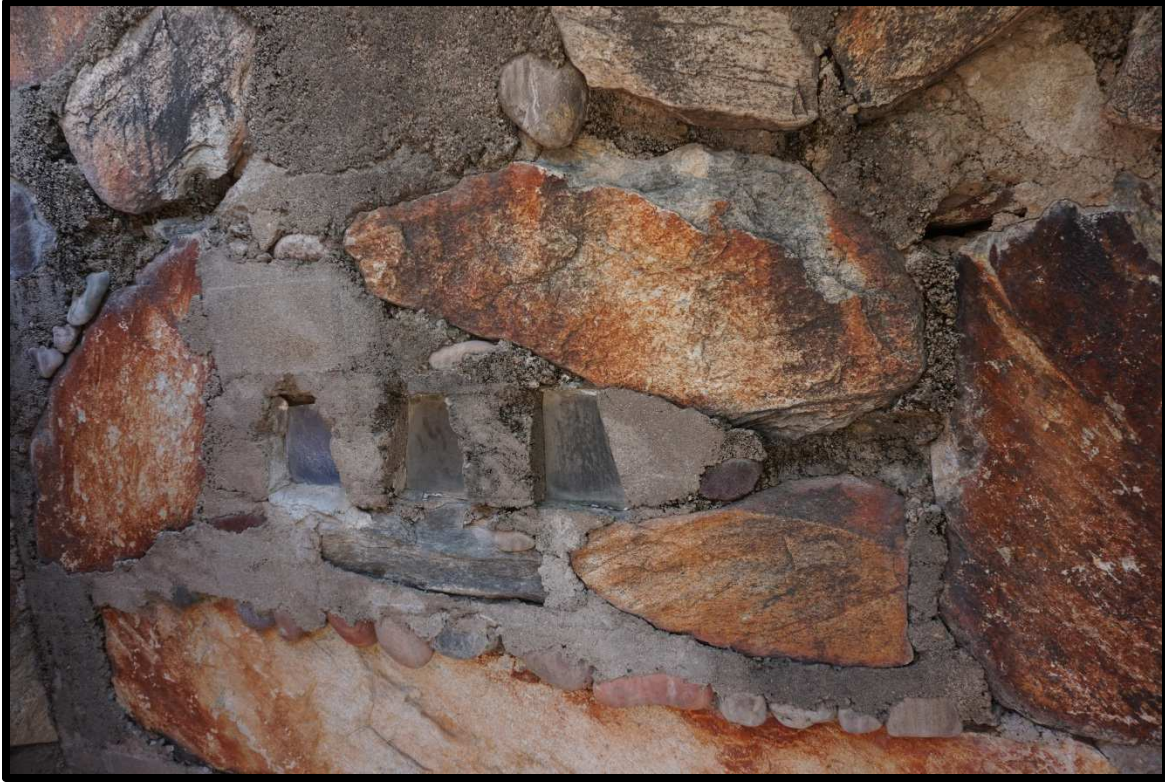
Figure 4.10. The Desert Masonry discovered in Wright's lab, Taliesin West; while the architect was experimenting with the techniques of using native materials.
