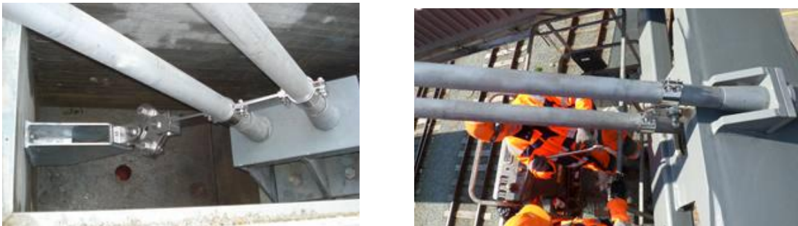
Figure 17 – Two models of Dampers installed in cable stay bridge in Denmark.
