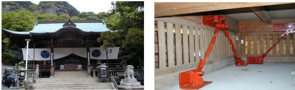
Figure 7 – Dampers with bracings installed in Yagurji Temple
