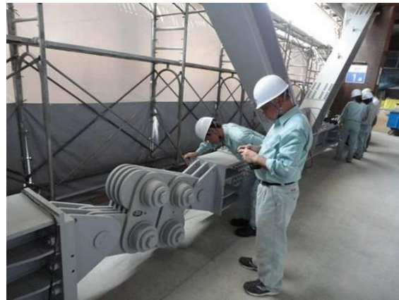
Figure 13 - 2250 kN Dampers installed for base isolation in the Abeno Harukas building
