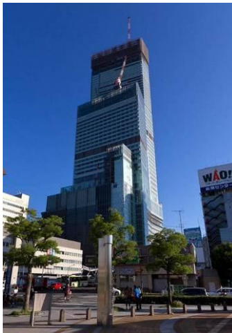
Figure 12 - Abeno Harukas October 2012 (under construction)
