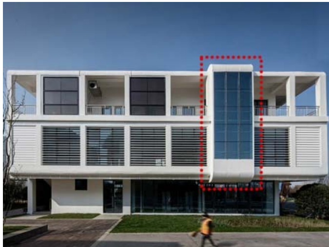
Fig.2. solar chimney in P+ building
