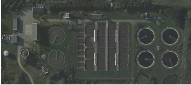
Figure 1: Kolding WWTP with two BioDenitro lines including four aeration tanks.
