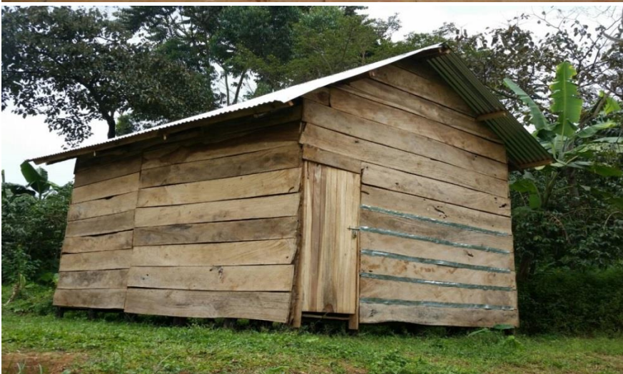
Figure 26: An improved low cost ambient ware potato store in Eastern Uganda
