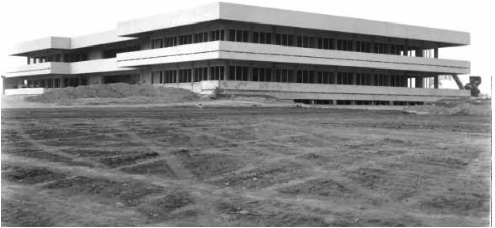
F.F. Hill, the Administration Building, also known as Building 500, circa 1977. Photo by IITA.
