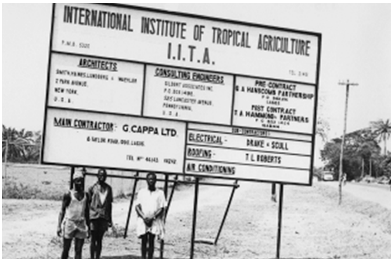
IITA entrance under construction in 1968.
