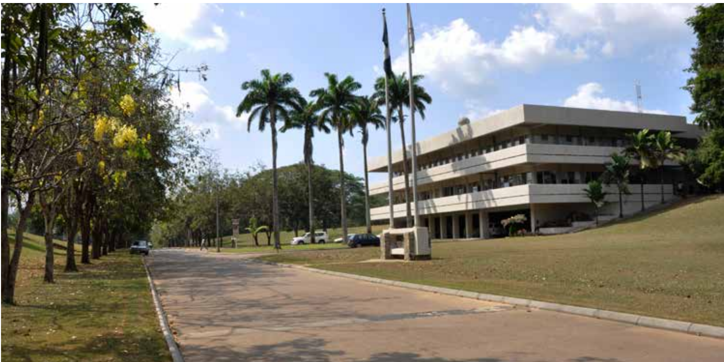
IITA Administration Building (Building 500) 50 years after.
