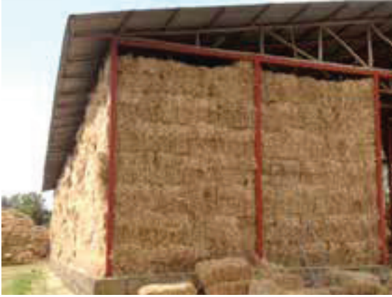
High roof hay store
