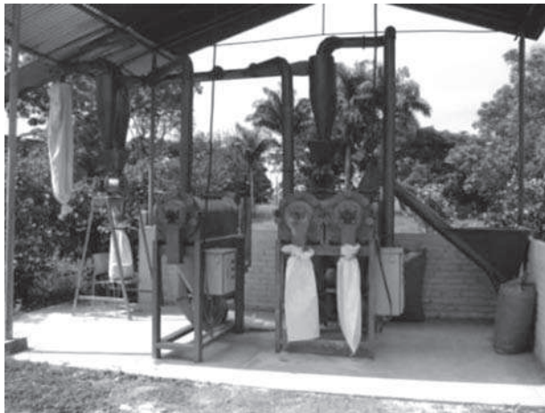
Figure 23-1. The CLAYUCA modular pilot plant for producing refined flour from dried cassava chips, Palmira.
