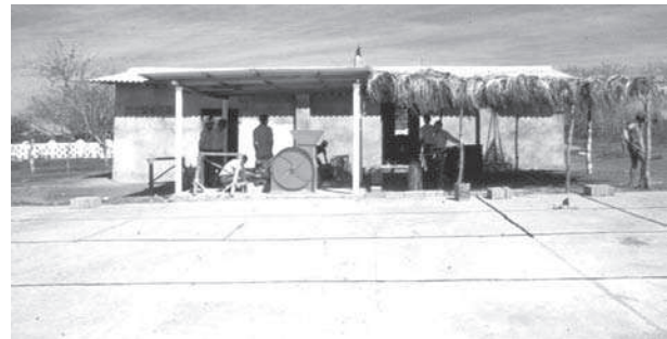
Figure 21-17. View of the roofing complex used to cover the cassava chipping machine and to protect the fresh cassava roots received for processing.
