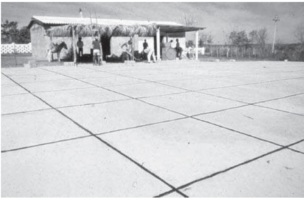
Figure 21-16. Final appearance of a drying concrete floor for cassava chips.
