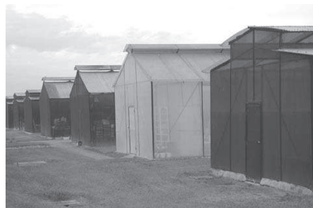
Figure 4-12. Screenhouse with a special mesh to prevent the transmission of viruses by insect vectors.
