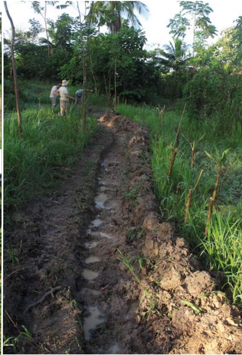
the undulating topography allows for recharge of ponds through a series of swales.
