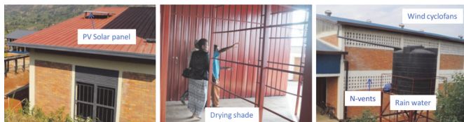
Figure 1. Features of demonstration drying hangars and warehouses built in the Eastern Province according to the climate-resilient guidelines developed by Climate-Resilient Post-harvest Agri-business Support Project (PASP) and ASAP. (Photographs were taken during assessments made in July 2016 by GEAR Ltd)
