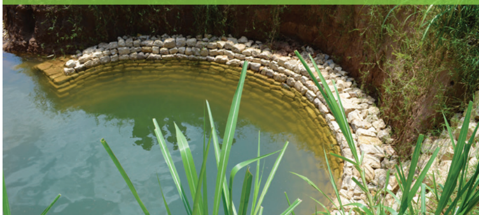
FIGURE 3. WATERSHED MANAGEMENT CAN QUICKLY IMPROVE WATER RESOURCES: A SHALLOW HAND DUG WELL IN ABRAHA-ATSBABA.
