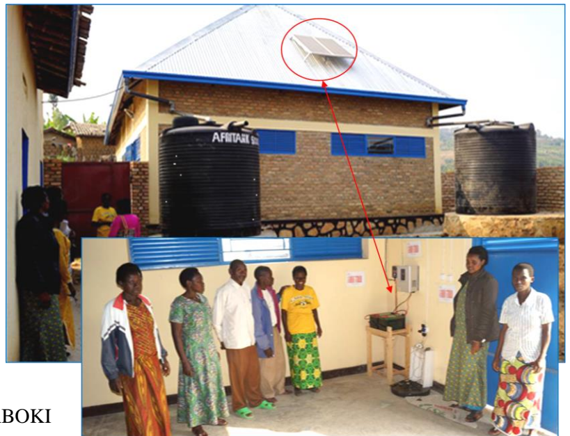
Figure 9 KOPABOKI cooperative, Kamonyi district: PHCRAB grant warehouse with rainwater harvesting and solar power, 12 th July 2016
