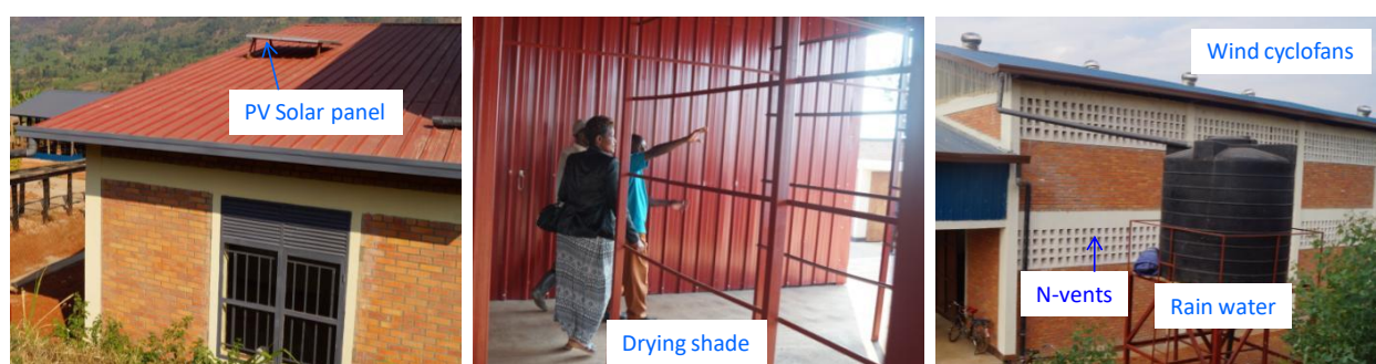
Figure 10 Features of demo drying hangars and warehouses built in the Eastern Province according climate-resilient guidelines developed by PASP-ASAP. Photos were taken during field work between 12 th and 22 July 2016.
