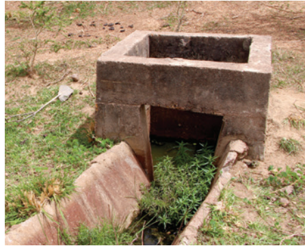
SMALL RESERVOIRS IN THE UPPER EAST REGION OF GHANA SHOWING (LEFT TO RIGHT) SILTATION, DYSFUNCTIONAL DISTRIBUTION CANALS AND DAMAGED IRRIGATION PUMP PIPES. SOURCE: BEDRU BALANA
