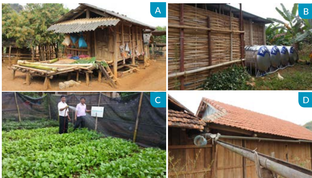
Photo 3.6 Harvesting rain to produce vegetables in Northwest Viet Nam. A: typical Hmong house in Thong village. B: the four tank units installed by WorldVeg/IWMI/FAVRI to store rainwater from the roof of a shed. C: vegetable garden irrigated with a rainwater harvesting system. D: traditional gutter made from bamboo sticks in Thong village. Photo credits: IWMI/Guillaume Lacombe
