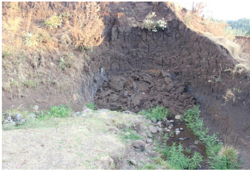
Photo 8: Soil slump and erosion of the upstream canals between the spring source and top of the Mush Irrigation Scheme canal
