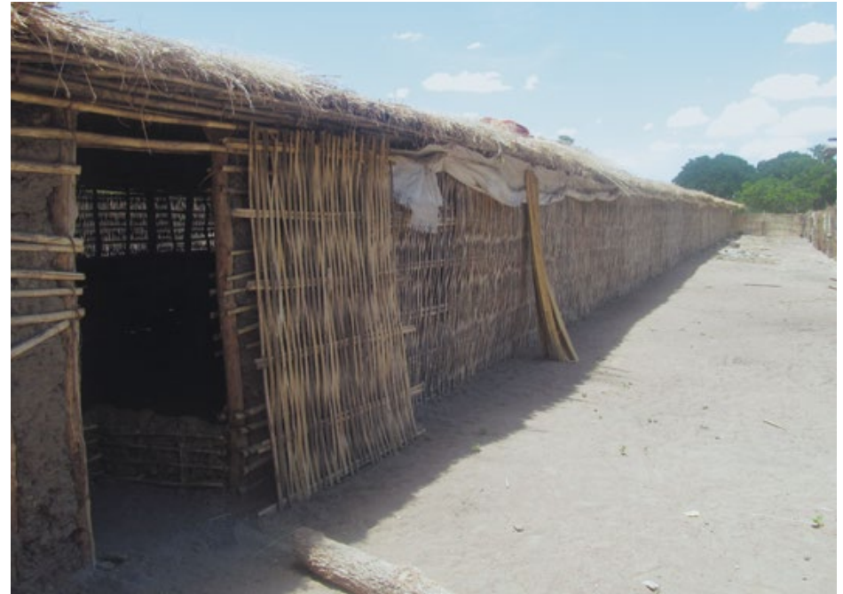
Side view of a broiler house
