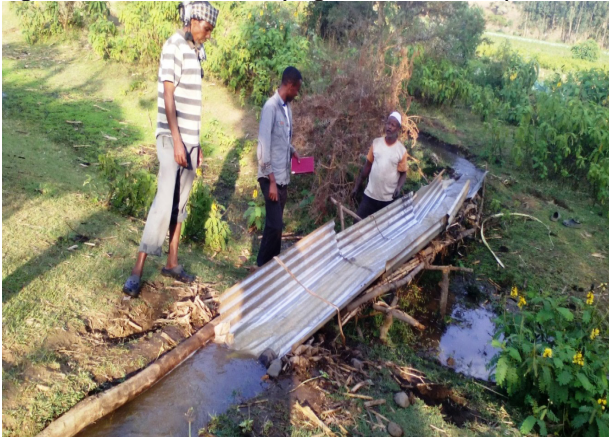
Figure 8. Method of conveying water over a depression at Waro scheme.
