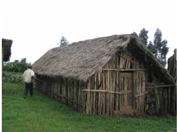
Ifoto ya 13: ubuhuniko bwinjiza umwuka n'urumuri muri Etiyopiya bwubakishije ibiti rusakajwe ibyatsi
