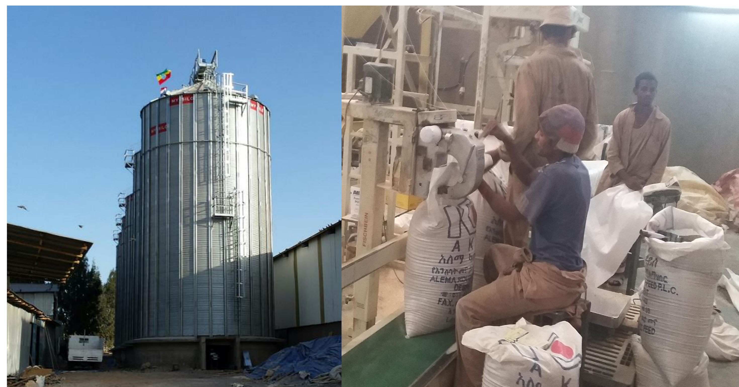
Grain storage (silo), animal feed processing, blending and packaging at AKF plant, Bishoftu, Ethiopia
