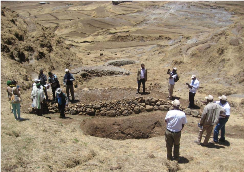
Percolation pits for water storage and irrigation use in Basona Worena
