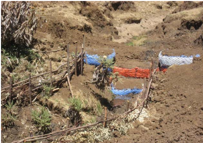
Gabions and gully shaping at the model watershed in Basona
