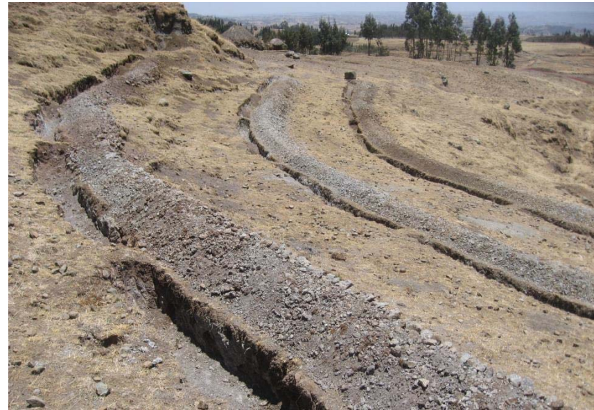
Partial view of trench structures for SWC and water retention at the watershed in Basona
