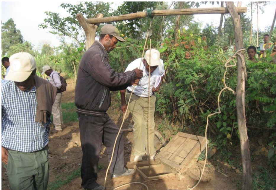
Shallow well with a pulley system to irrigate vegetables and avocado trees
