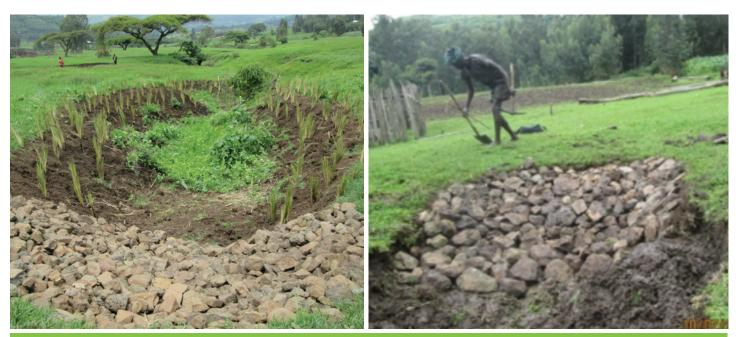
PICTURE 2: GULLY HEAD TREATMENT USING STONES OF DIFFERENT DIAMETERS (PHOTO: MESERET B. ADDISIE)
