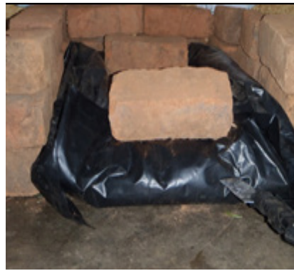
Picture 8: Bricks keeping the polythene in place. Knife slits on the bottom edge to let effluent drain.
