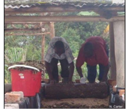
Picture 6: Using a log to compact a layer
