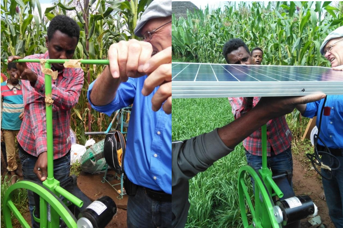
Figure 3: Installation of solar pumps and fixing the solar panel
