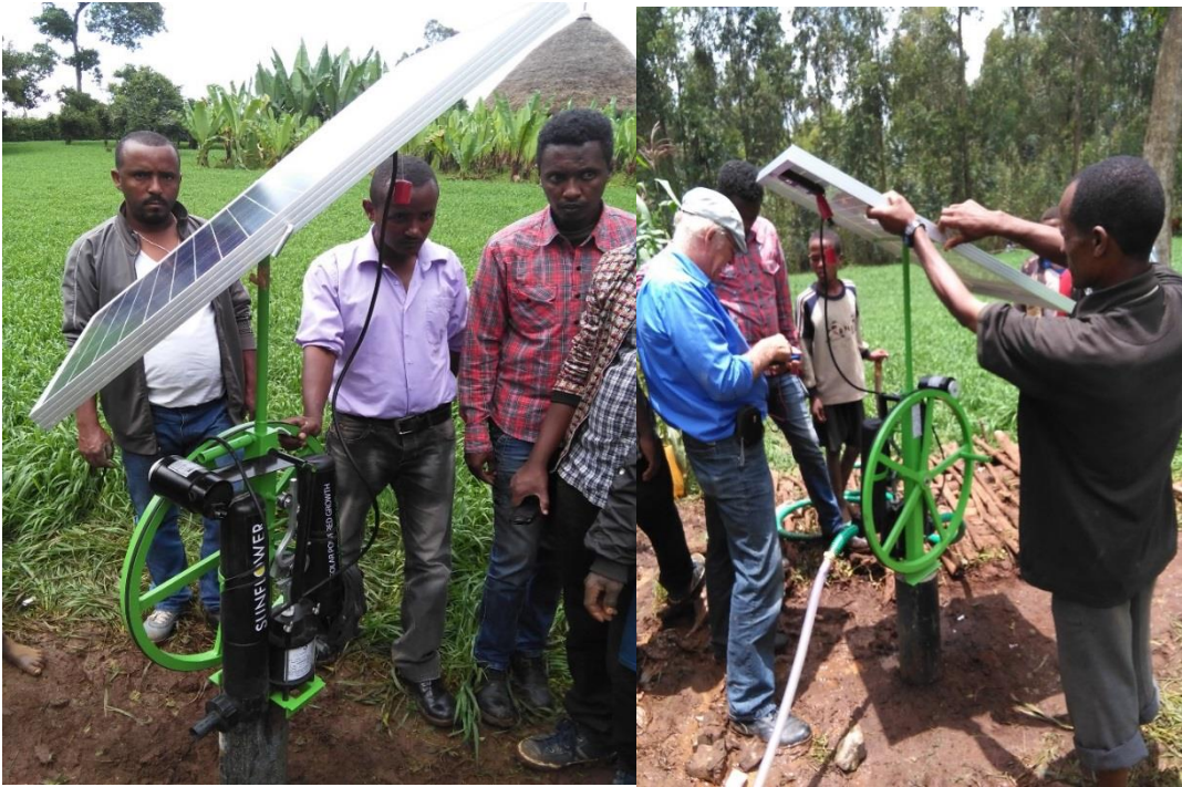
Figure 4: Installation of solar pumps and the solar panel
