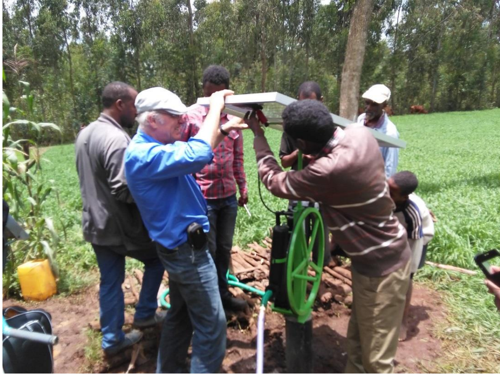
Figure 5: Demonstration about the installation of solar pumps
