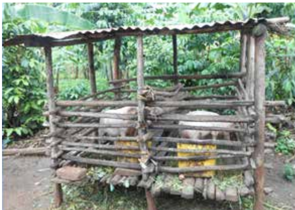
A raised house with wall and floor made of wood and iron sheet roofing—Masaka.
