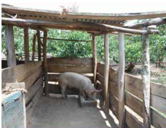
A non-raised house with cement floor, timber walls and iron sheet roofing—Mukono.
