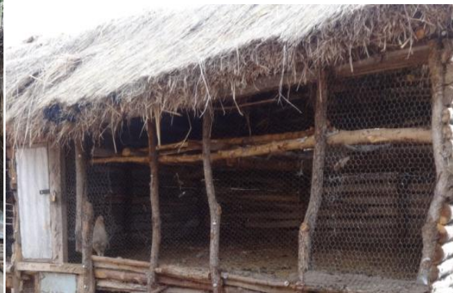
Figure 8: Traditionally roofed poultry shelter, but prone to wind and cold
