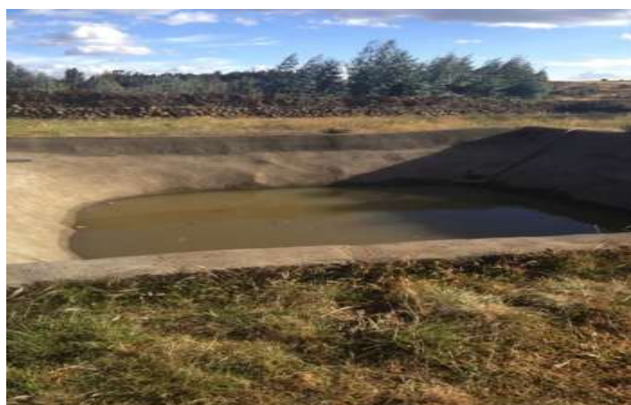
Photo 2: Water harvesting at Workjur of Denjan village, Gosh Bado kebele
