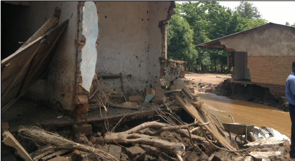
Photo 4: House washed away during flood, February 2014 T/A Mlolo, Nsanje district Photo credit: Augustine Tonde.
