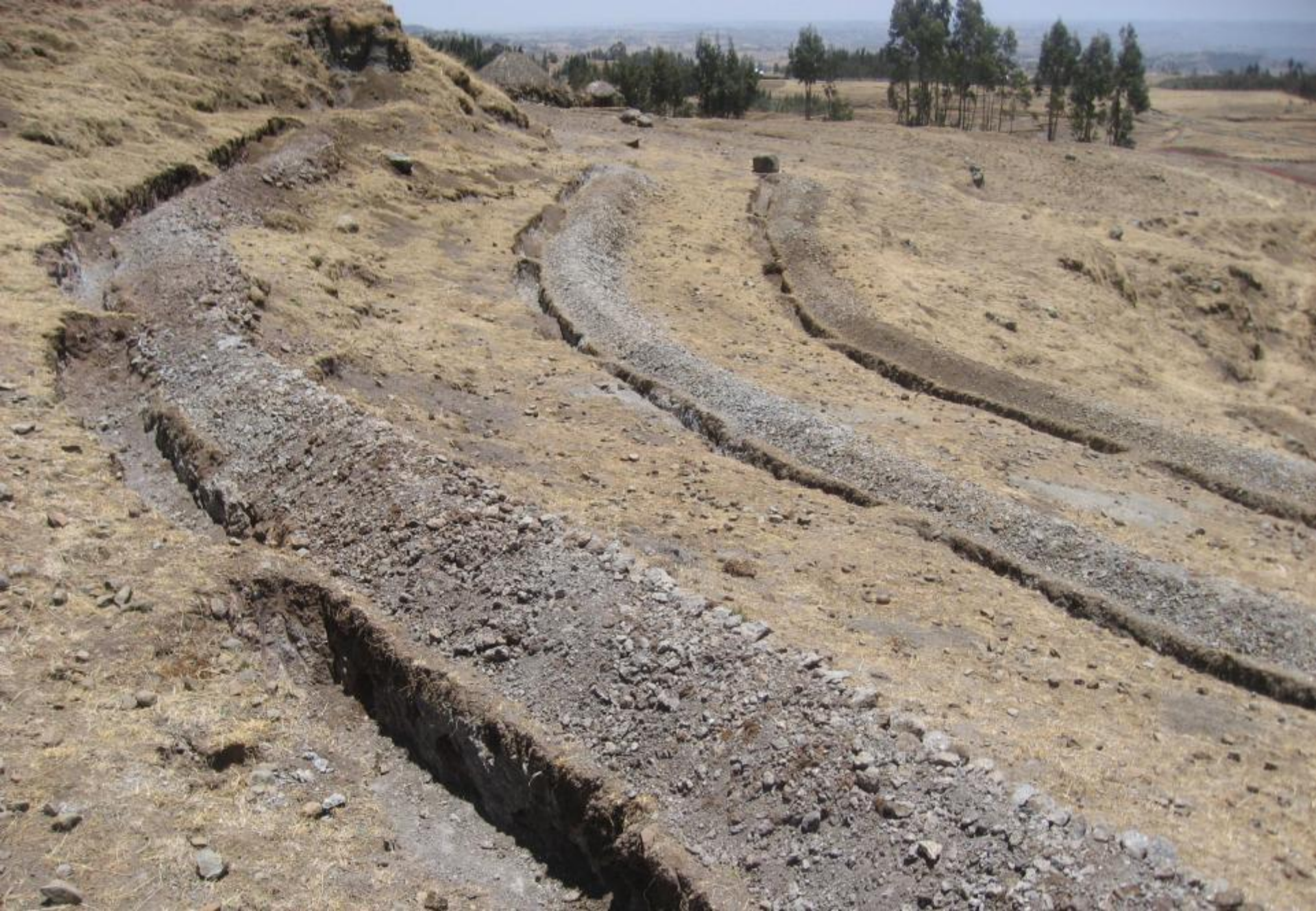
Partial view of trench structures for soil and water conservation and water retention in Basona Worena
