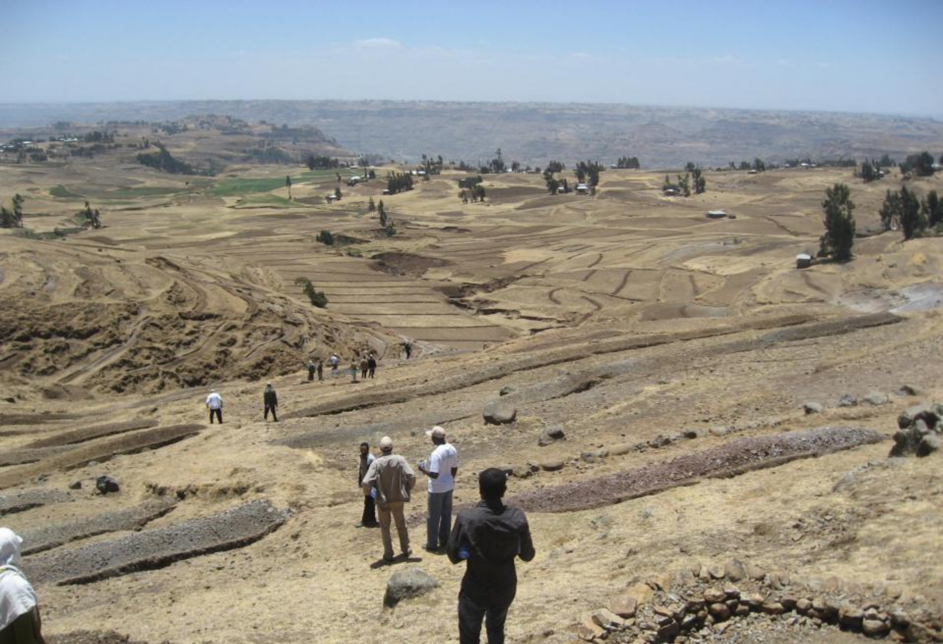
Soil and water conservation and water harvesting structures in Basona Worena
