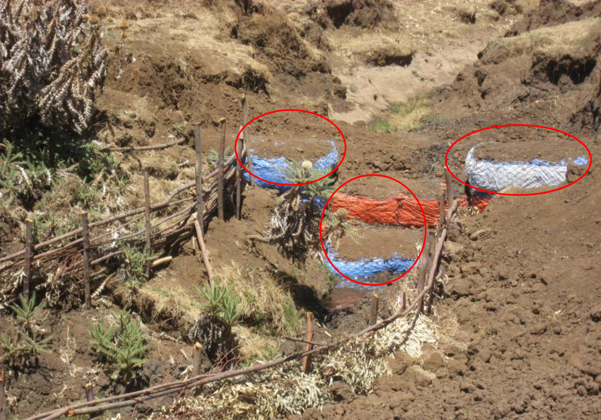
Gabions and gully shaping at the model watershed in Basona Worena
