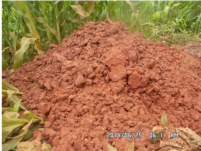
Picture 2. Brown soil excavated out to increase depth of a well from 3 m to 3.36 m in Upper Gana.
