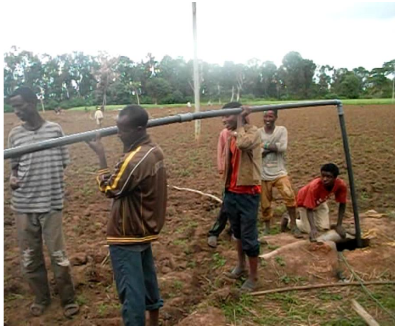
Picture 5. Existing well protection style observed which is exposed to erosion, flooding and contamination.
