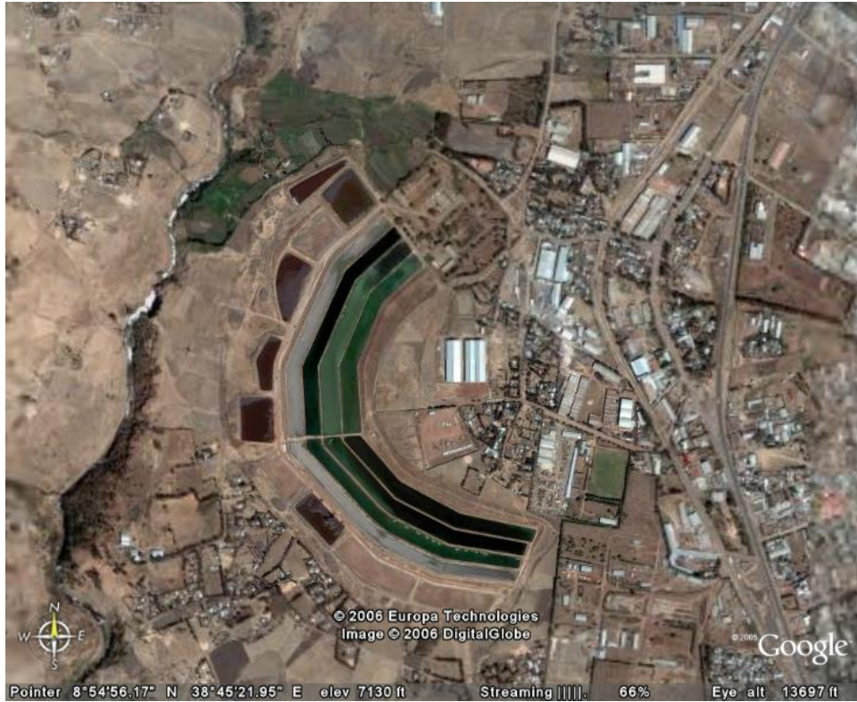
Figure 2: Kaliti Oxidation Pond: The modern sewer treatment plant in Addis
