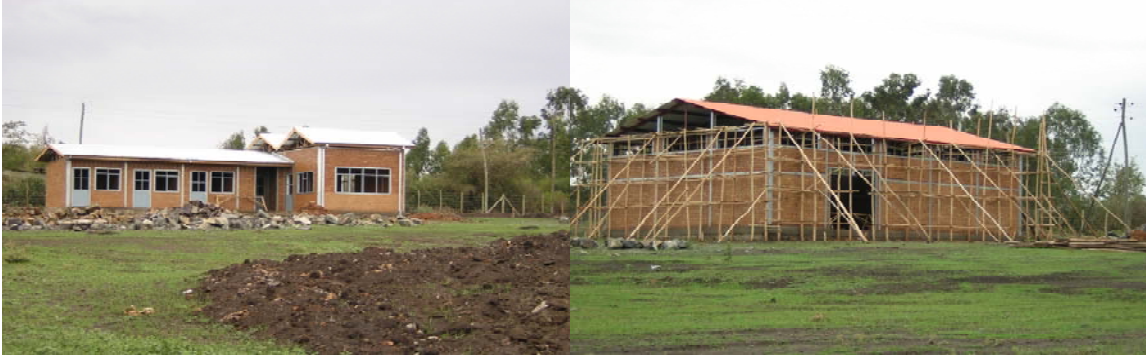
Figure 4: The new cooperative office and milk processing plant under construction
