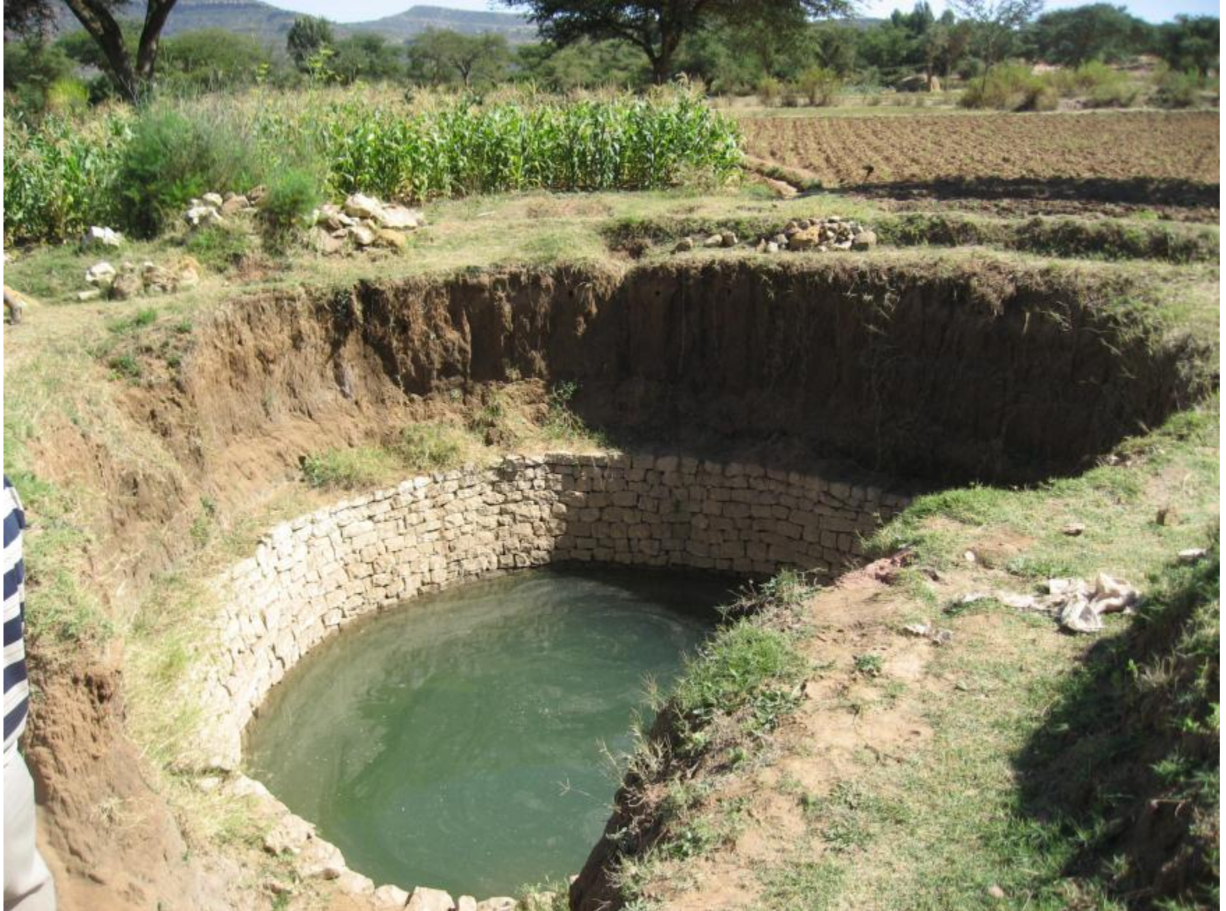
Wells developed as a result of IWM (gully rehabilitation, hill side restoration, enrichment planting, construction of trenches and check dams) - used to irrigate and grow food crops and fruit trees
