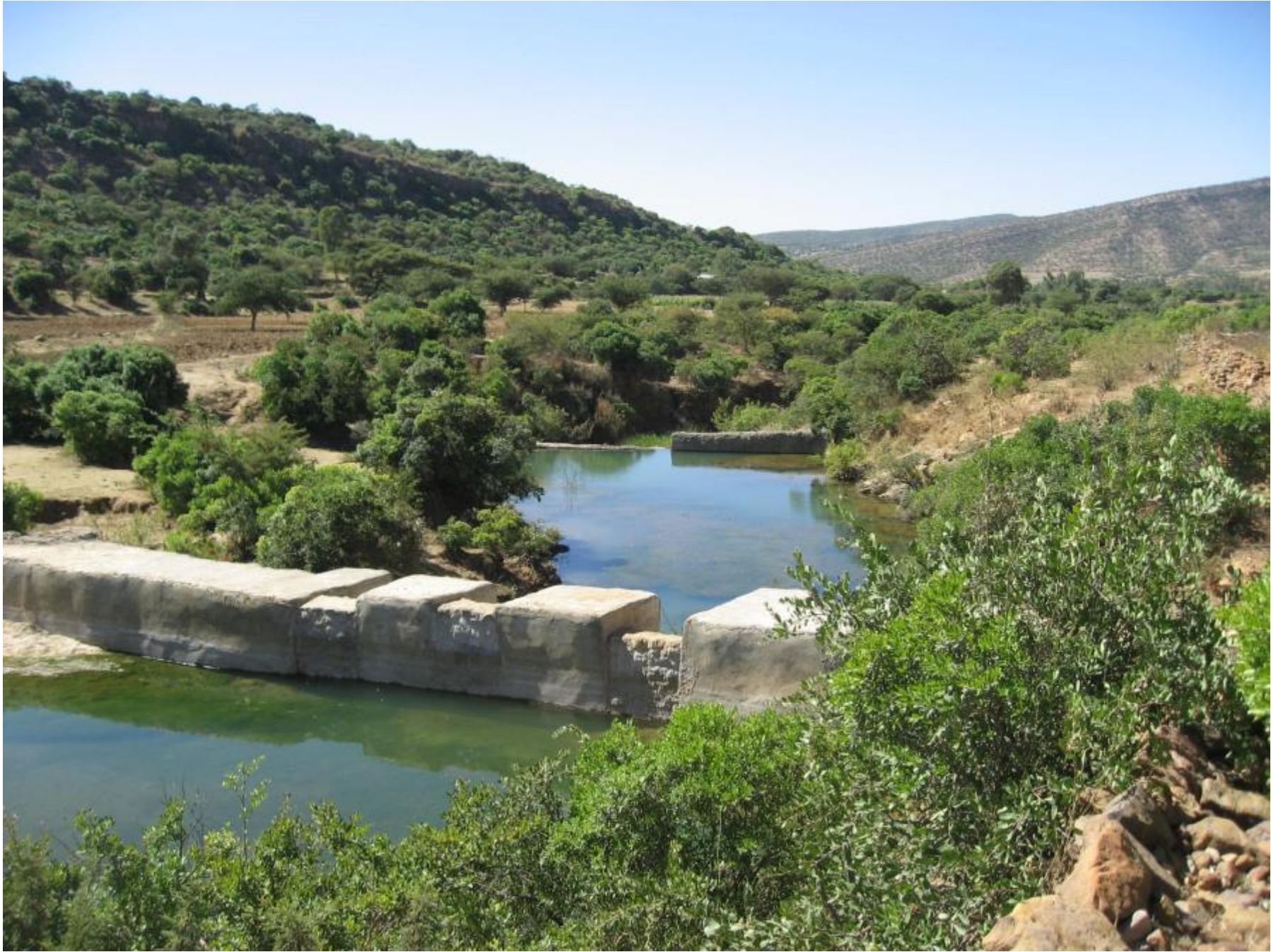
Check-dam ponds constructed by communities for multiple uses in Abraha Wa-Atsbaha, Tigray
