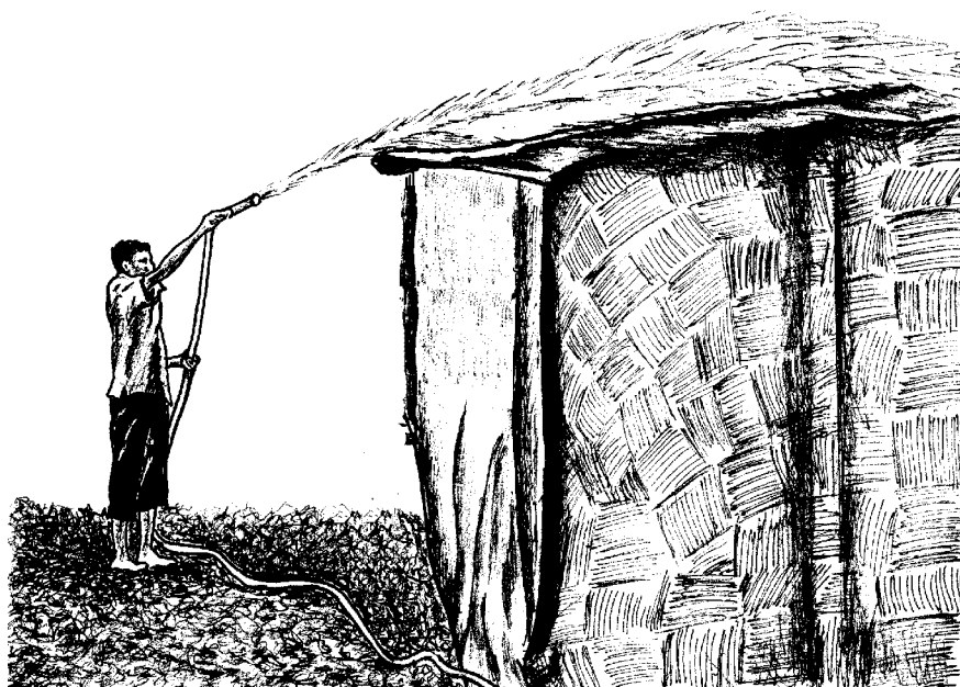
Figure 26: Spraying the jute-covered roof
