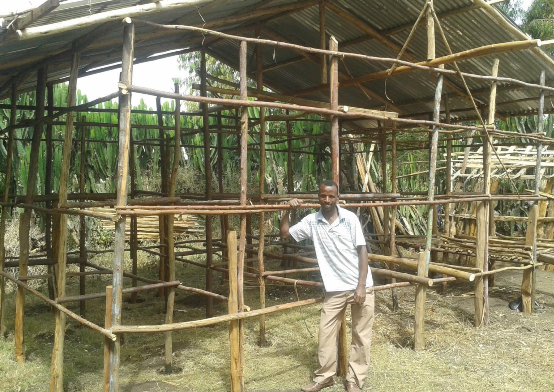
Sinana (Oromia): Diffuse Light Store (DLS) construction
