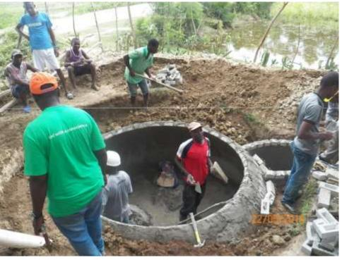
✓ Built on a circular concrete base
