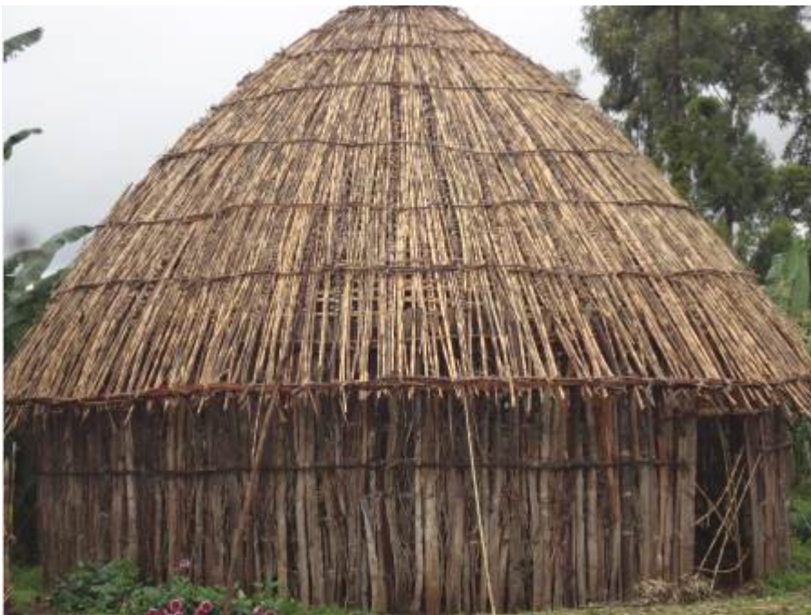
Figure 26:: Bamboo poles for thatching and Eucalyptus timber for house construction
