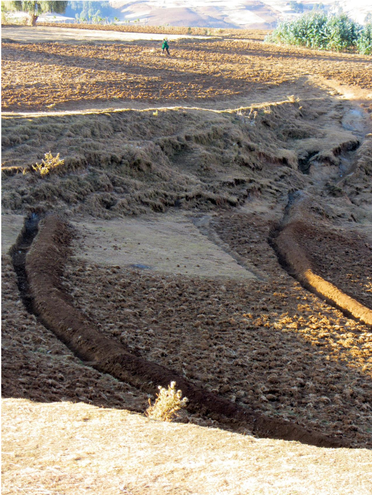
Soil conservation work, Jeldu
