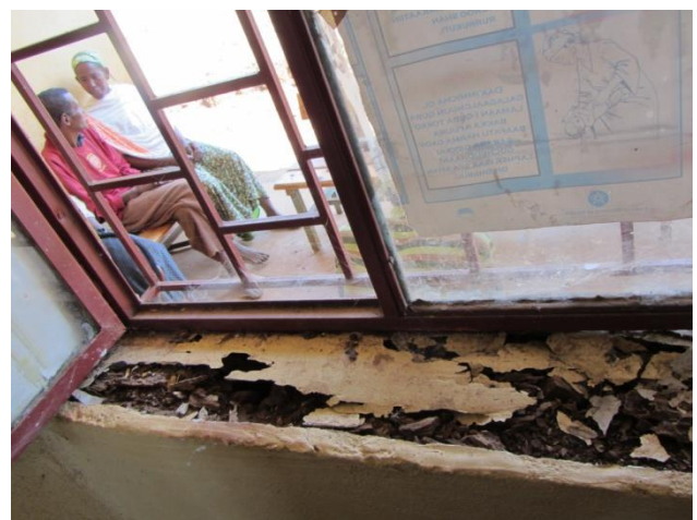
Termite activity and destruction of newly built health station in Bikila
