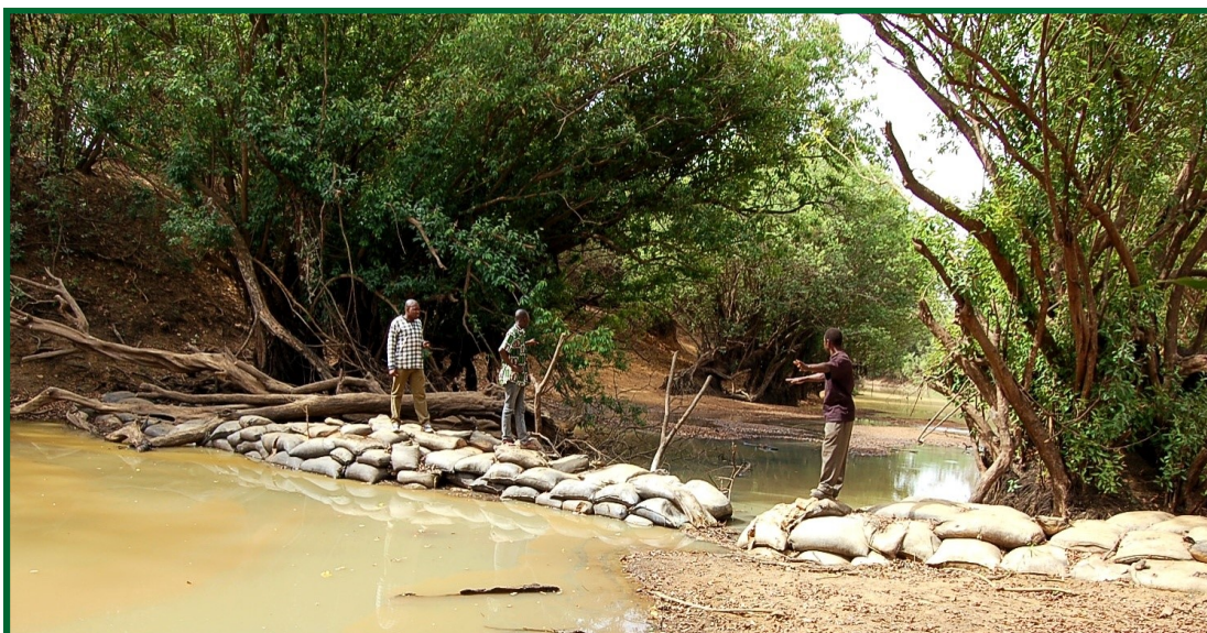
Ouattara Lassina, Diébougou fisherman (right), shows Aly and Joachim how the fishermen , on their own initiative, tried to dam a portion of the Bougouriba river to create more water for fish during the dry season. A man who lost his watch among the sandbags broke the dam (V4, Burkina Faso).
