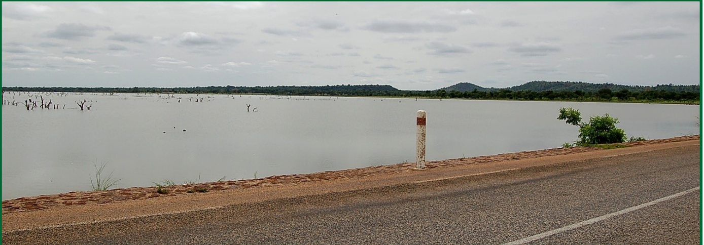
The highway between Diébougou and Gaoua creates the Bapla dam and large reservoir (V4, Burkina Faso, June 2012).
