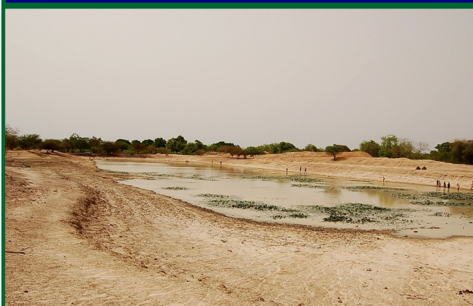
This dugout near Yako, Burkina Faso, was dug through a project. A nearby community uses it to water livestock. At the beginning of the late 2013 rainy season, it is not yet full (V1 PGIS, June 2013).
